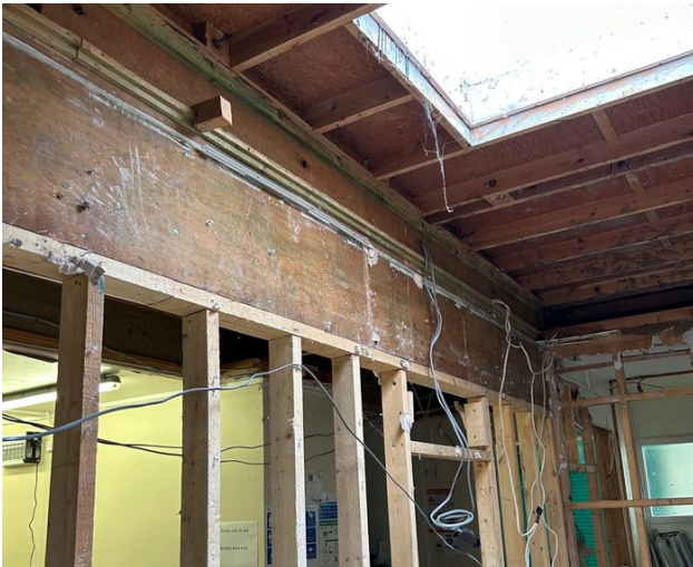
Before: the old kitchen stripped back, ready for structural and M&E works
