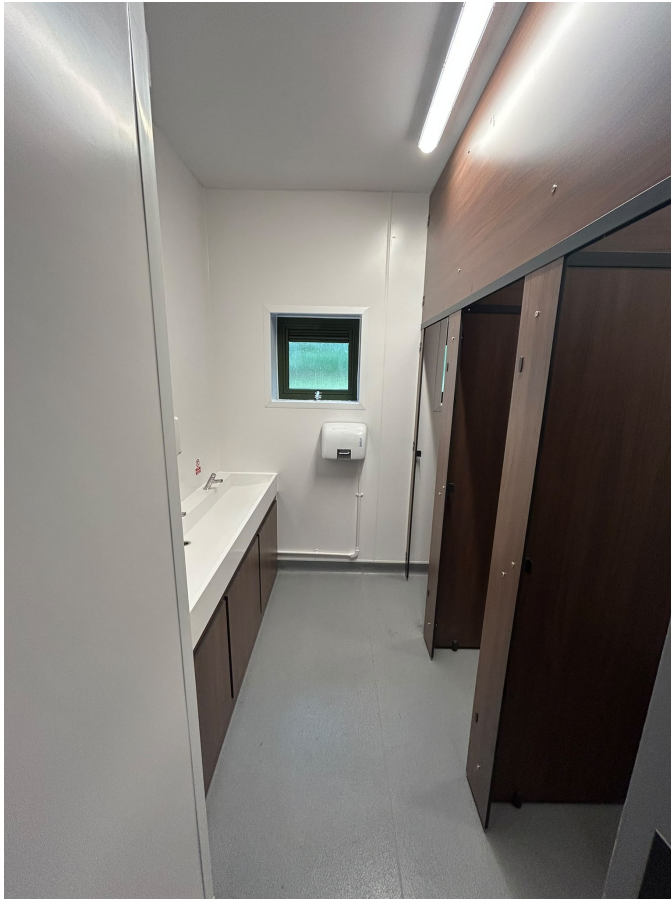
The refurbished washroom, with new trough basin and toilet cubicles
