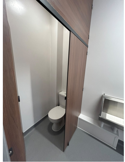
New WC cubicle and stainless steel urinal
