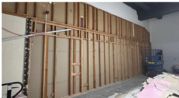
Demolition on night shifts
