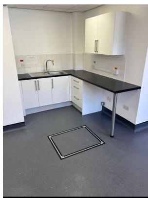
Staff facility upgrade
