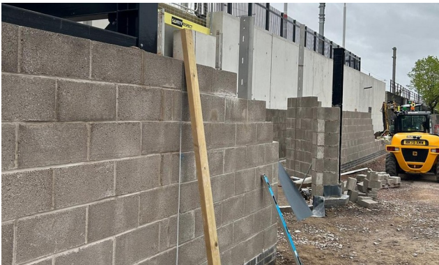
Before: blockwork backing walls ready for cladding
