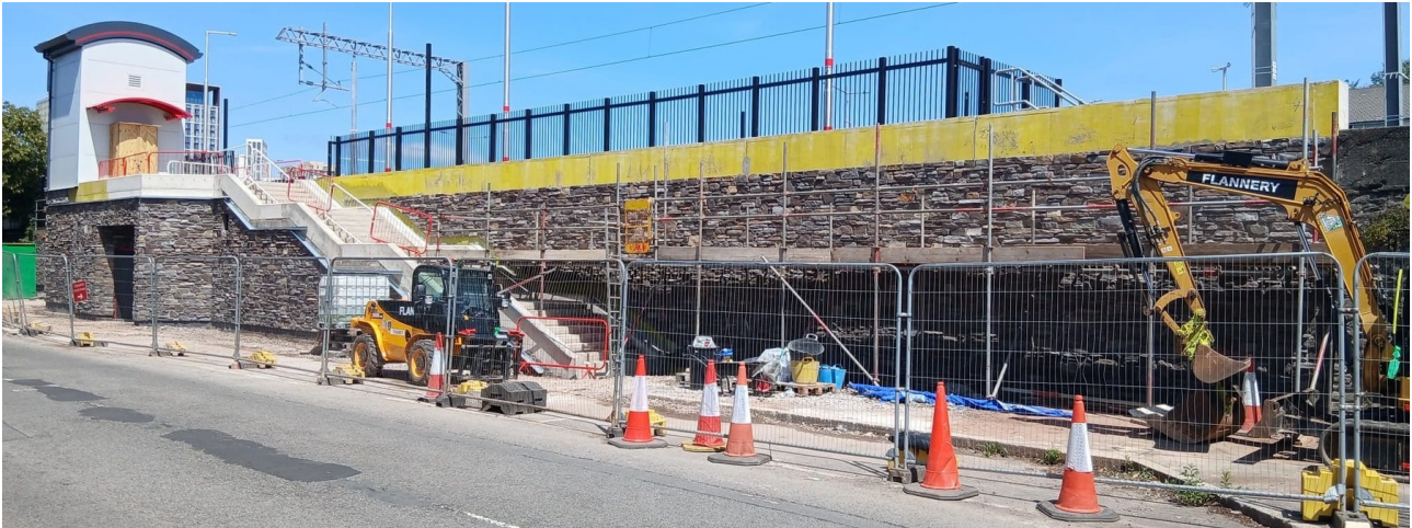
Stone cladding to the Bute Street retaining wall, worked from scaffold alongside the lift and stair tower
