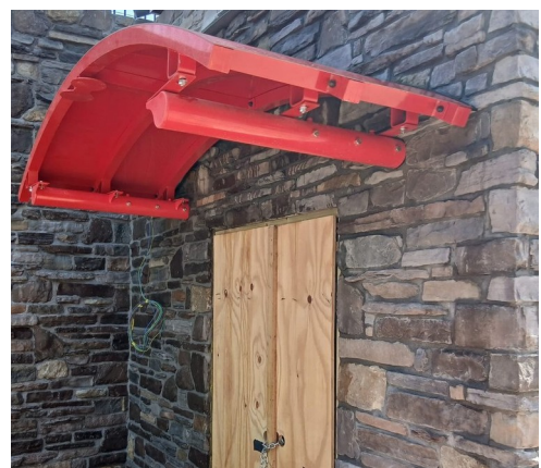
Stonework around the canopied entrance
