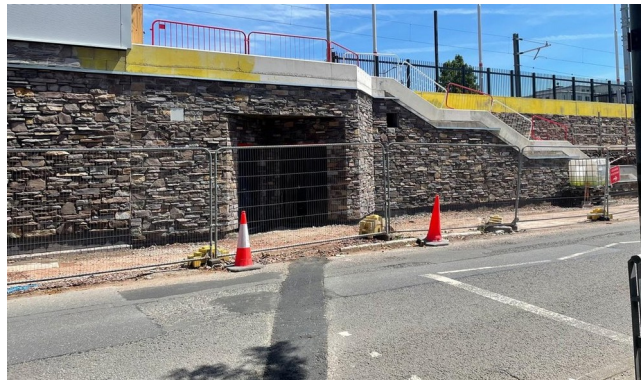
After: completed stonework to the entrance elevation
